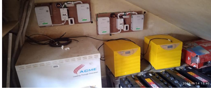
Wheeling to the Grid
